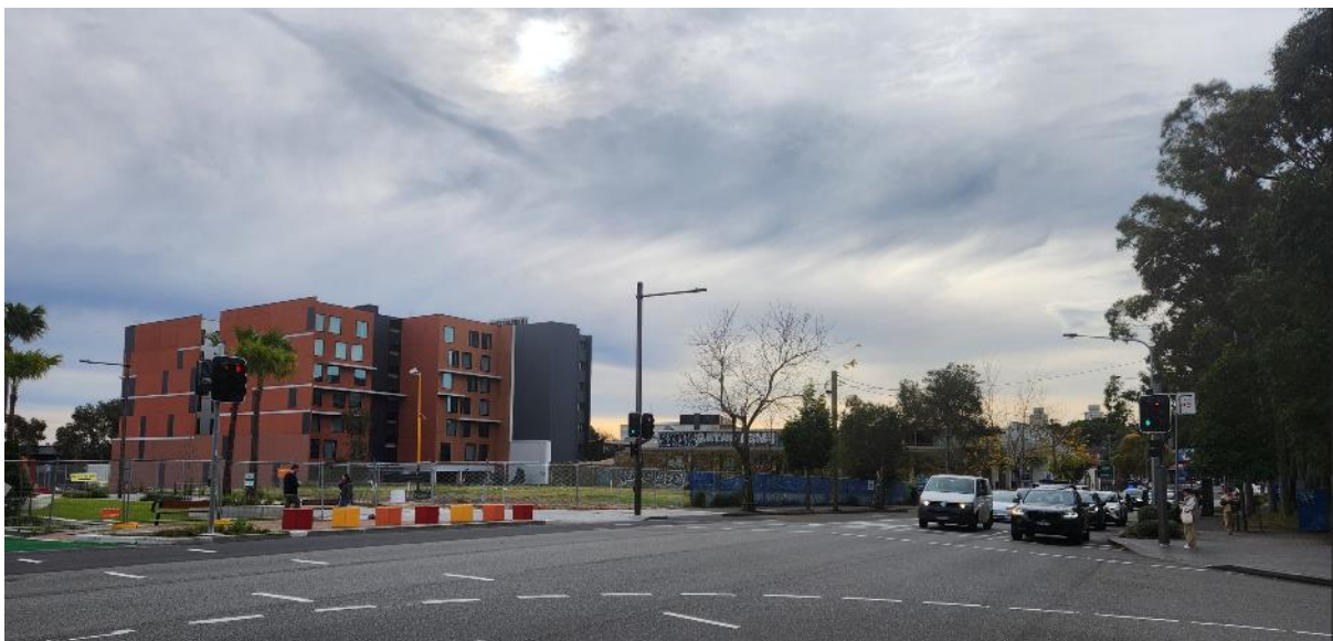
Figure 11: View looking north west from intersection of Botany Road and Geddes Avenue
